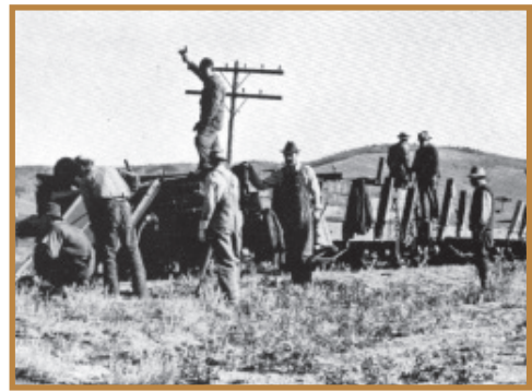
With the "end of the line", a scrap train crept along with a winch on the first car used to pull the rails up a ramp and onto the flat cars. Photo by R.H. Kindig, Colorado Rail Annual No.12.
